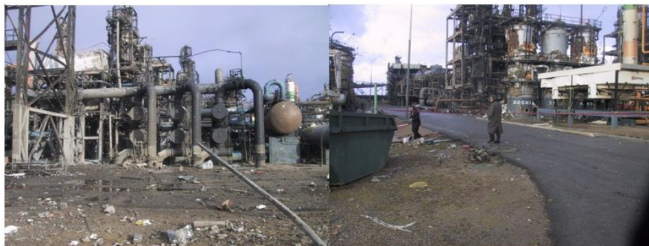
Figure 1. Damage caused by the explosion of GNL Skikda on June 20 th , 2004.
